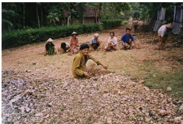
Community in Yogyakarta control site maintaining intra-village road
